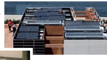
The "intelligent roof" has three different types of solar collector, which can be separately deployed to meet the energy requirements of the house at any one time
