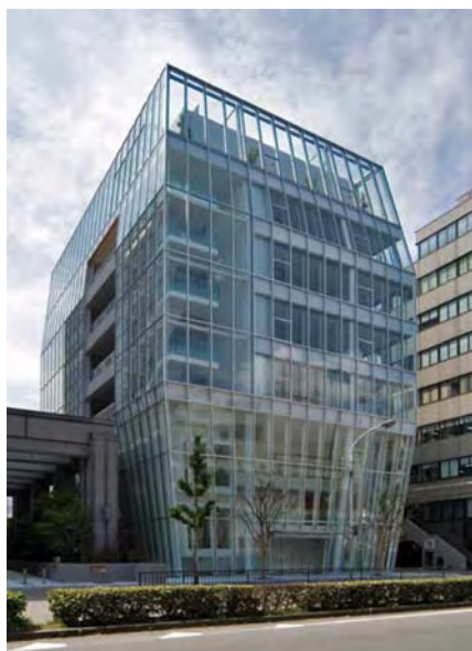
Kyoto Head Office opens annex.
